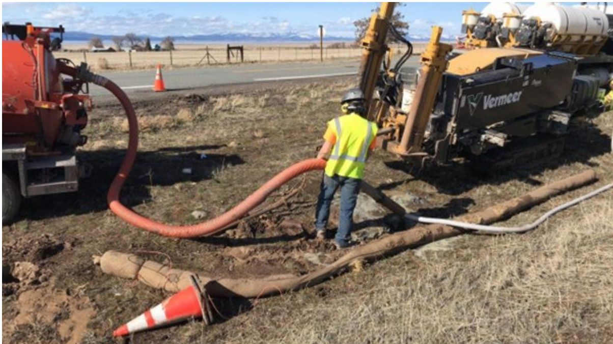
Photo 3: Overview bore location with conduit. Clean-up post pull back of conduit.
