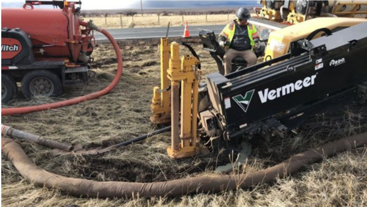
Photo 1: Overview bore hole insertion.
