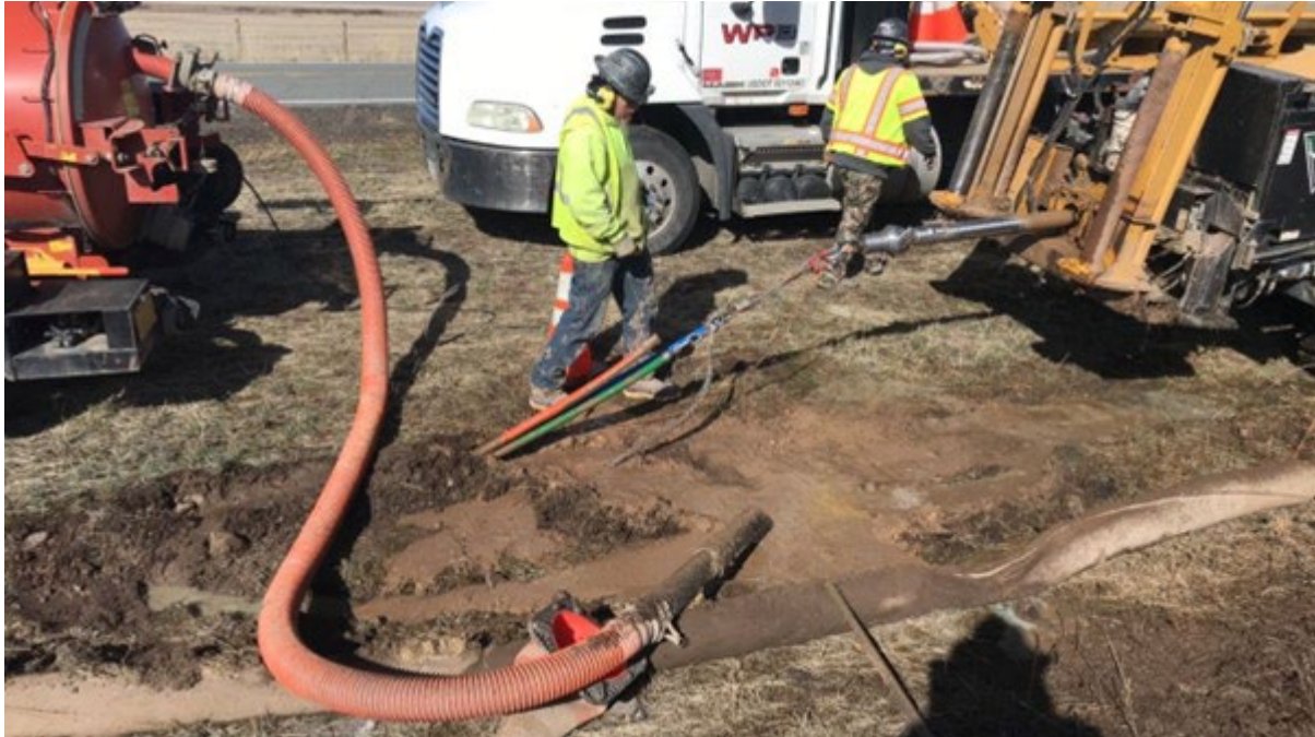
Photo 2: Overview Bore location with conduit pulled back.
